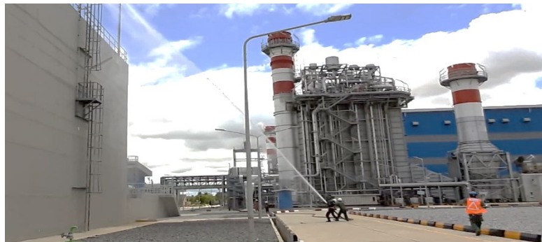
Emergency Response exercise for in case of fire at Water Treatment Plant – PERT Team mobilization
